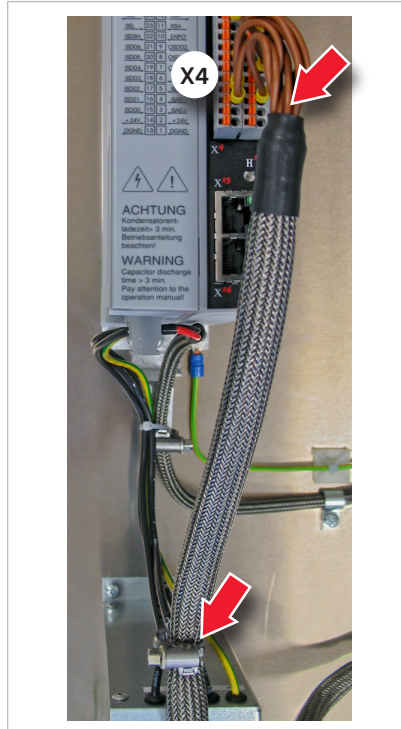
Illustration 18.2 Specimen setup - Detail 4: Control cables
